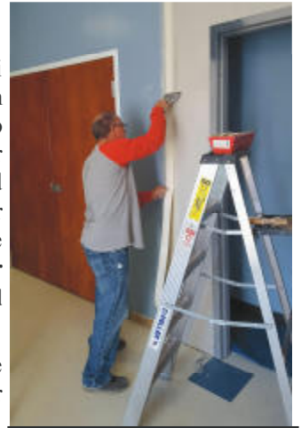
Ken May finishes drywalling the closet addition.
